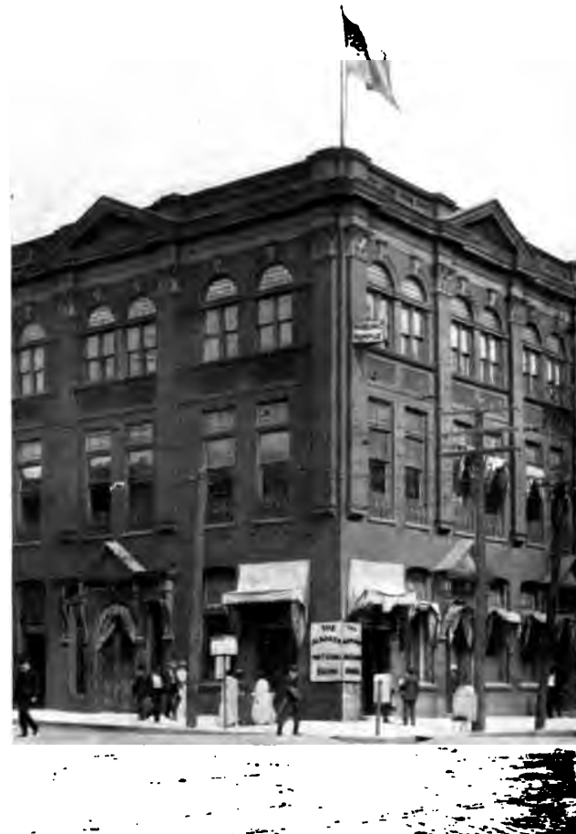
ALABAMA NATIONAL BANK, Birmingham, Ala.
